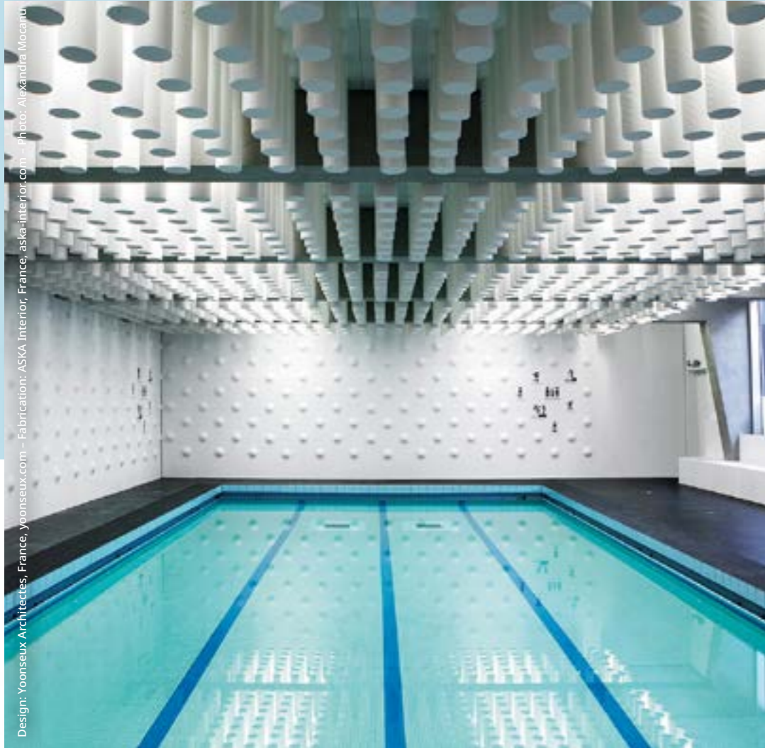
Thermoformed wall-claddings in one of Paris' coolest indoor pools.
